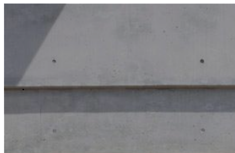
CPC3 Decorative profile finish concrete precast spandrel, natural concrete finish with grey oxide.
