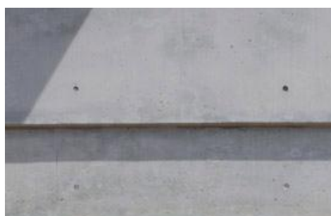
CPC2 Decorative profile finish concrete precast spandrel, finish to match COF1
